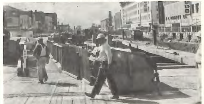
Temporary decking over subway construction.
