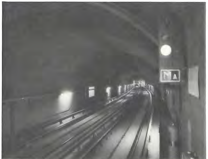
Tunnels on the Metro are lighted all the way for safety and comfort. Note the signal (upper right) that provides the train operator with indications about the track ahead.
