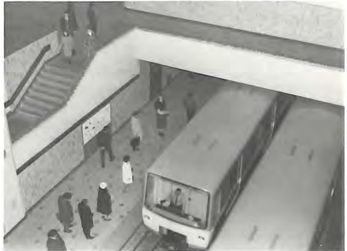
This view of CREMAZIE looking down from an open mezzanine conveys the feeling of free and uncramped movement.
