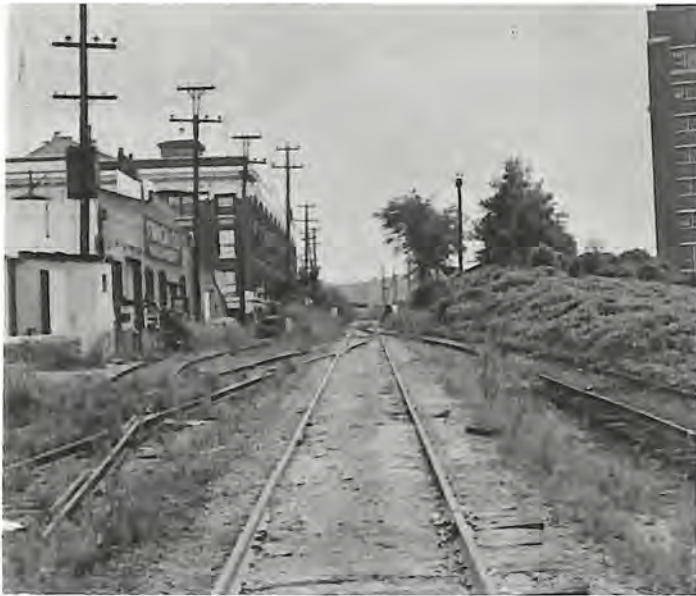
Southern Railway line looking south toward Ponce de Leon Avenue bridge at Sears. The many side tracks and spurs must be kept in service; this creates a problem for either busways or rapid transit, the solution of which is complex, costly, and time-consuming.
