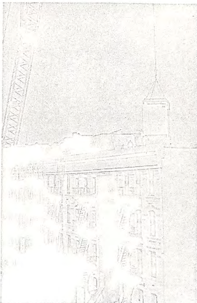
Moments later, unit is lowered toward roof of the building for which it is destined, an unoccupied old-law tenement in which a hole has been made from the roof down.
