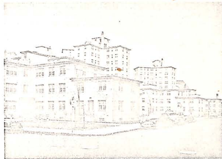
High and Low Buildings . . . Harold F. Kellogg; Thomas Worcester, Architects
