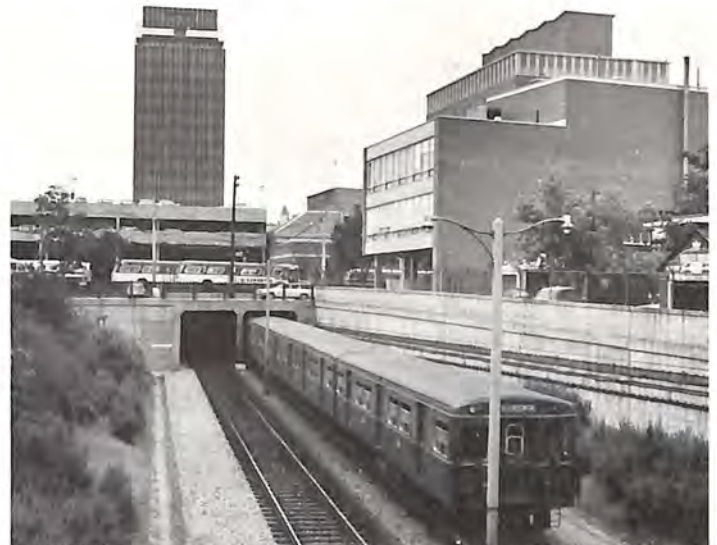
Rapid Transit train approaching Eglinton Station with high-rise building and parking decks using “air rights” over tracks.
