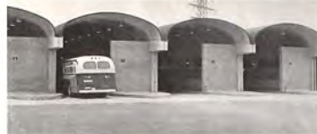
Toronto makes good use of "Bus 'n' Ride" service. Buses circulate through residential areas, pick up hundreds of thousands of people each day, and deliver them to a nearby subway station for completion of their trip downtown.
