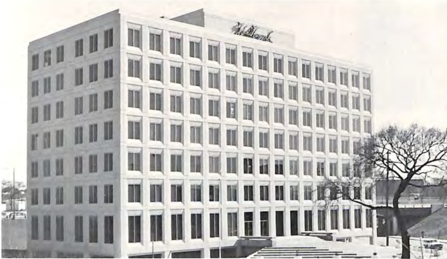
John Hancock Building – Butler Street
