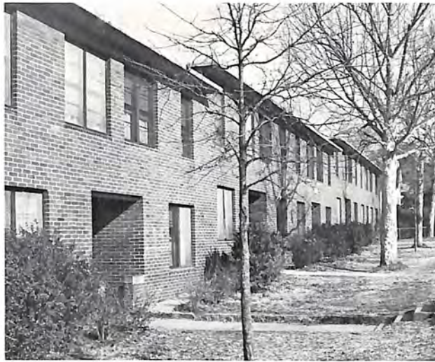
1941 / ALONZO F. HERNDON HOMES—CONSTRUCTION ON THE last of three of Atlanta's low-rent housing developments completed in 1941 were the Alonzo F. Herndon Homes. These 520 units added substantially to the city's ever-growing need for low-rent housing. More than 2000 people live in this near-downtown area of the city.
