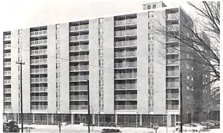
JOHN O. CHILES HOMES — a 250-unit project, with 222 apartments in a 10-story high-rise building and 28 garden-type apartments . . . adjacent to Joel Chandler Harris Homes . . . with 272 tenants . . . average age 71 . . . average monthly rental $28.50.
