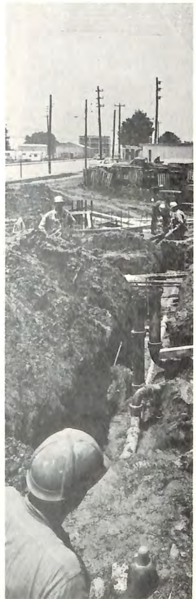
McDaniel Street construction
