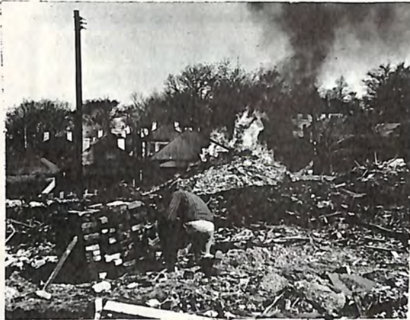
Park site demolition
