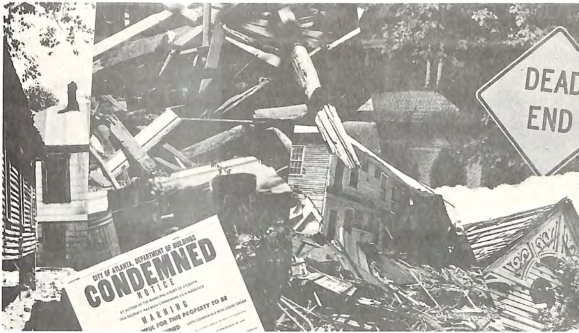
ONE OF THE great community benefits of urban renewal is the removal of unsafe, unsanitary and inadequate buildings.
