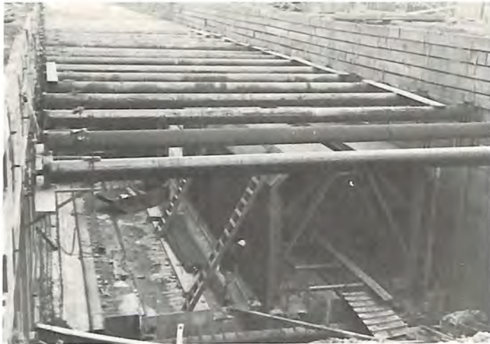
Subway construction in Oakland; steel form for subway shell in place on right.
