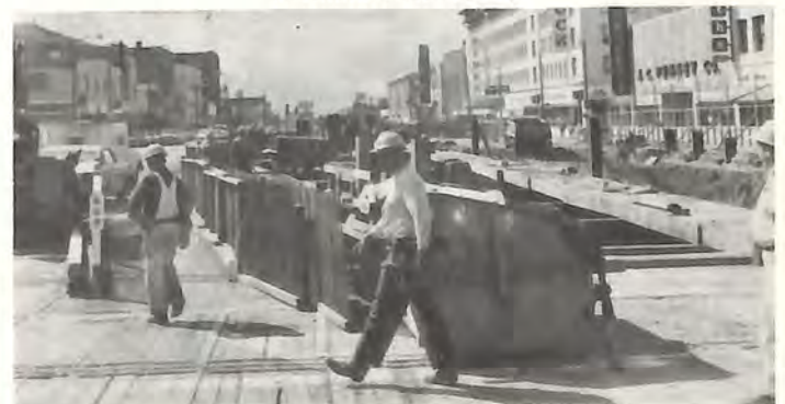
Temporary decking over subway construction.
