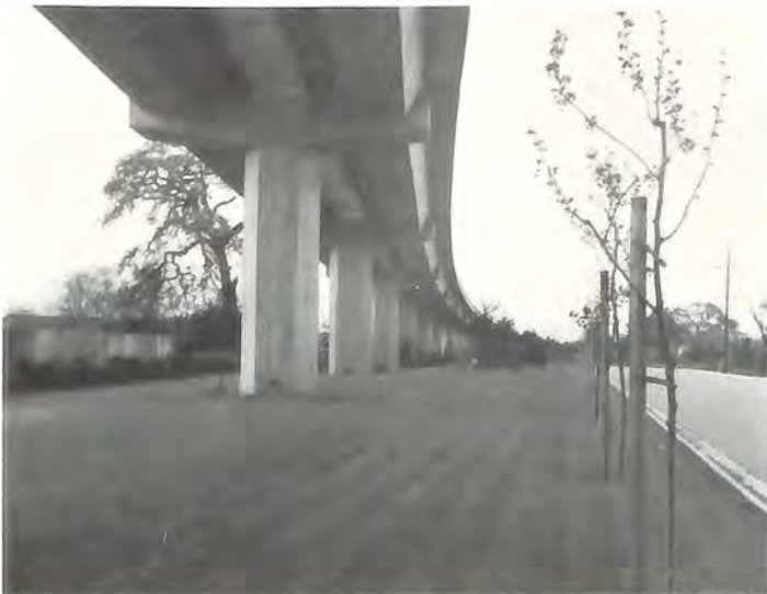
Completed section of aerial structure, with landscaped "linear park" beneath.
