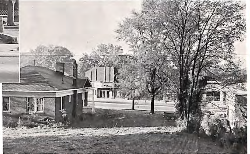
View at right shows rear of building and big area suitable for parking. Lot runs back 300 feet from street.
