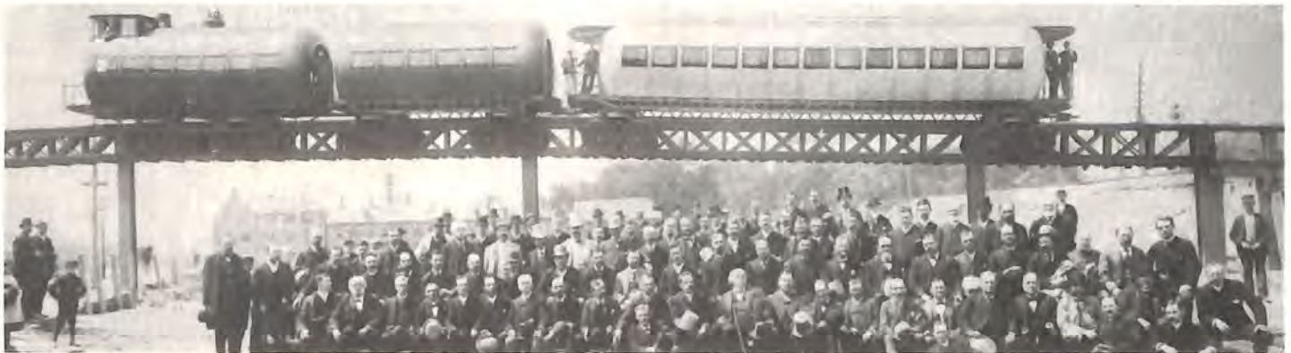
MEIGS COLLECTION, Yale University Library — MONORAIL, 1887 VERSION — Joe Vincent Meigs (second row, sixth from right) patented this early "monorail" in 1873. The running wheels were tilted at 45 degree angles; horizontally-mounted steam-driven wheels running on an up-
