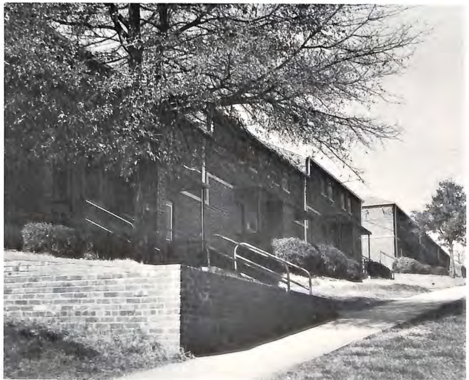
1953 / CARVER COMMUNITY— WITH THE TERMINATION of World War II, and in a city where thousands of returning servicemen were seeking a place to live, the first post-war project of the Atlanta Housing Authority was completed. Carver Community, a development of 990 units with more than 4500 residents, is adjacent to shopping conveniences, schools and many commercial facilities.
