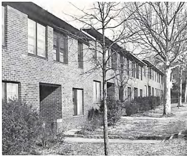
1941 / ALONZO F. HERNDON HOMES—CONSTRUCTION ON THE last of three of Atlanta's low-rent housing developments completed in 1941 were the Alonzo F. Herndon Homes. These 520 units added substantially to the city's ever-growing need for low-rent housing. More than 2000 people live in this near-downtown area of the city.
